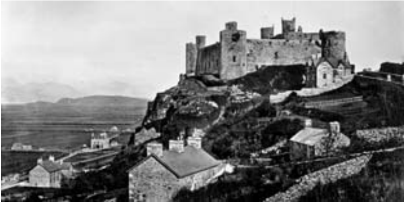
Figure 20. Harlech Castle, Wales. This early photograph shows the castle before modern restoration and encroaching buildings. A fortress gatehouse (upper right), curtain walls, and corner tower plus the remarkable site enabled the castle garrison to withstand sieges until they were starved into submission. The sea once came up to the base of the cliff; the flat land at the left and the area occupied by the road and houses would have been under water. Gramstorff Collection, Photographic Archives, National Gallery of Art, Washington, DC.
