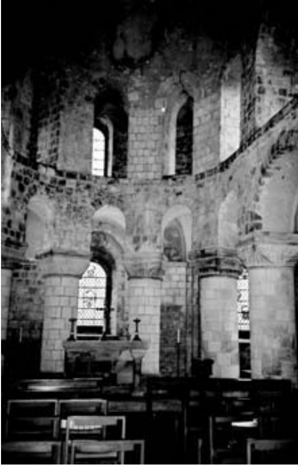
Figure 9. Chapel of St. John, Tower of London, interior. An arcade on massive round piers divides the space into a nave and side aisles. The second-story gallery opening into the nave continues around the entire tower and provides access to the gallery from the principal rooms. Photograph: Anna Leider.
