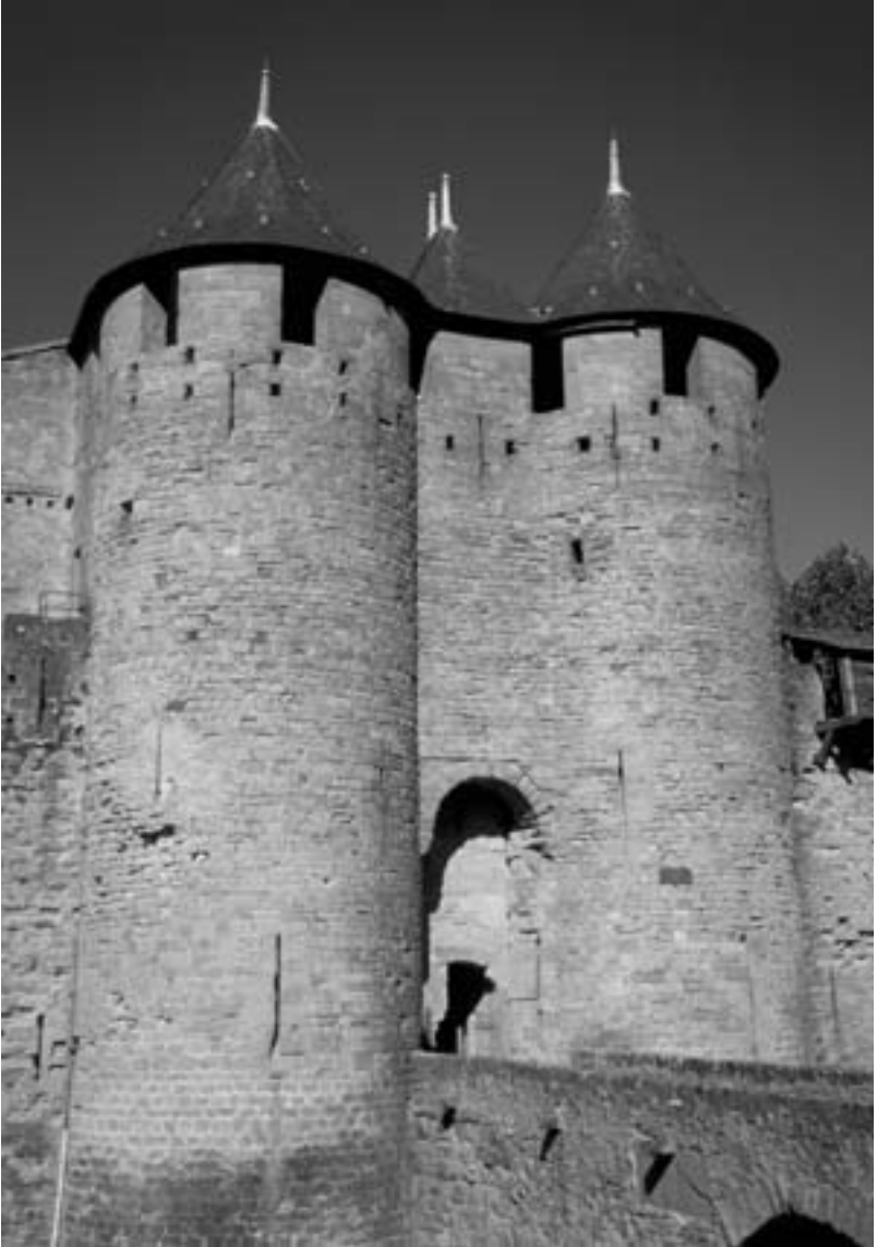
Figure 11. Castle of the Counts, Carcassonne, France. Although the entrance into the Castle of the Counts is within the fortified city, it has independent defenses, including a ditch once crossed by a drawbridge and a pair of round defensive towers. At the top of the crenellated towers, holes for the ends of beams supporting wooden hoardings can be seen. Photograph: Karen Leider.
