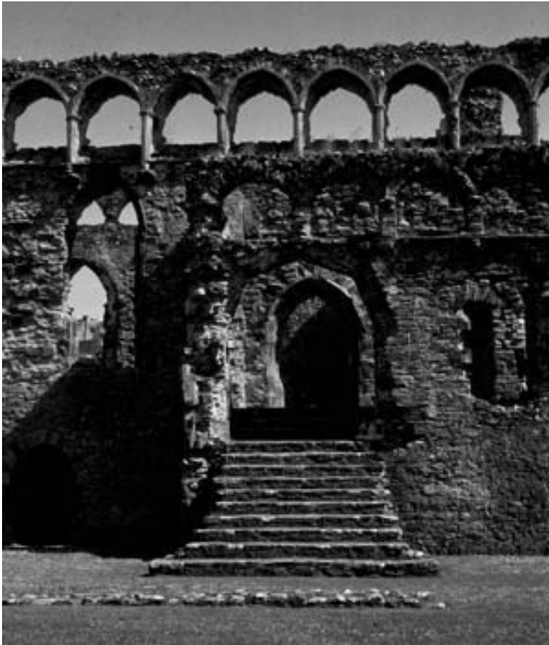
Figure 25. Grand stair, Bishop's Palace, St. David's, Wales. Few of the grand palatial stairways still exist, but the Bishop's Palace boasts of two. The normal medieval stairway was an unimpressive and often difficult tight spiral fit into the wall of the building. Photograph: Karen Leider.
