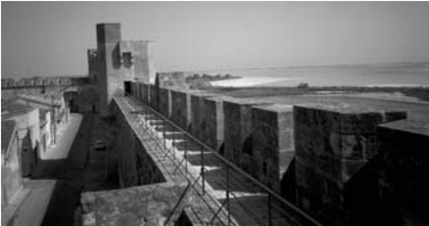
Figure 22. City walls, Aigues Mortes, France. Founded as a port for crusaders in the thirteenth century, the city has relatively low walls and many gates that once provided an easy access to the ships. The top of the wall has a wide walk and crenellations tall enough to protect the guards. To prevent treasonable tunneling, no houses were permitted next to the walls. This space also enabled soldiers to move rapidly into defensive positions. The tower at the left is one of the fortified gates. Photograph: Marilyn Stokstad.
