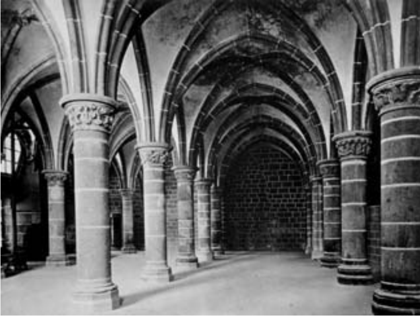
Figure 18. The Knights' Hall (scriptorium); Mont St.-Michel, France. The work-room, or scriptorium, where books were copied and illuminated, in the monastery of Mont St.-Michel was built in the first decades of the thirteenth century. The room suggests the appearance of the great halls once found in castles and palaces. Columns with carved capitals support a ribbed groin vault and divide the space into bays. Tapestries could be hung to form semiprivate compartments. Large windows and fireplaces provided light and heat, and two garderobes were additional amenities. Gramstorff Collection, Photographic Archives, National Gallery of Art, Washington, DC.
