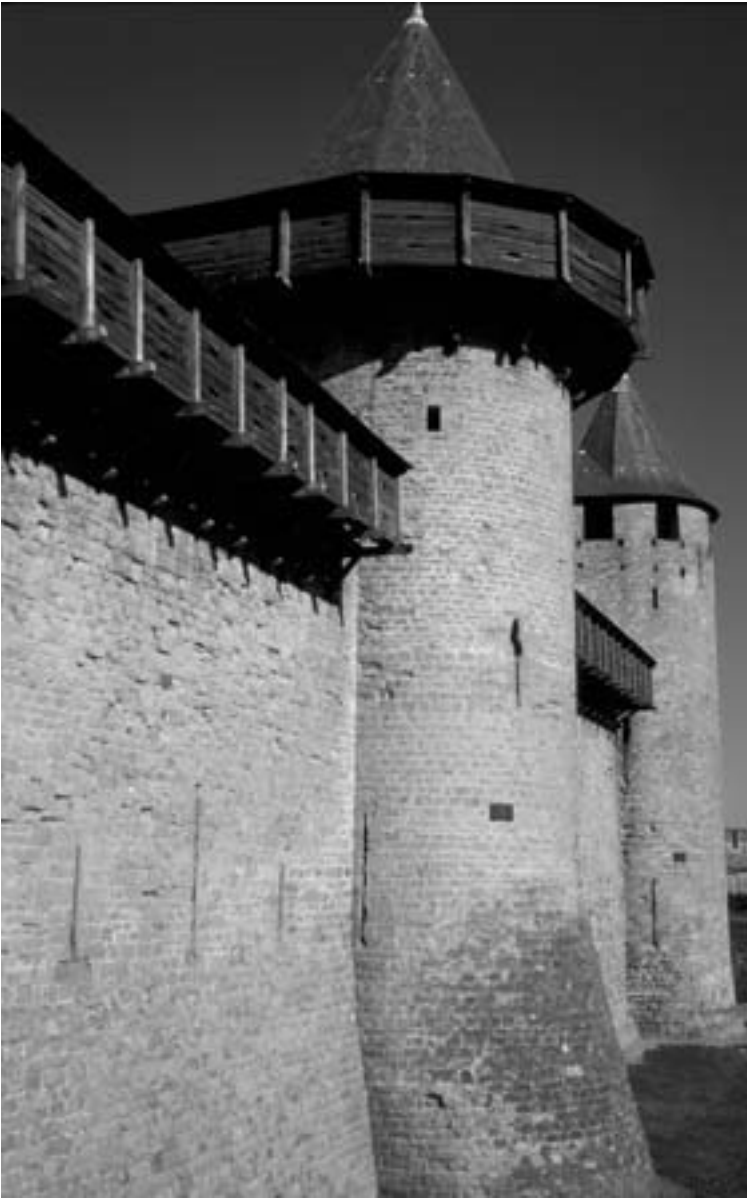
Figure 12. Wall and towers with hoardings, Carcassonne, France. As restored by Viollet-le-Duc, this section of the walls represents the city as it would have been seen when prepared for war. Hoardings were temporary wooden platforms and walls that doubled or tripled the space available for the defenders on the top of the walls. Photograph: Karen Leider.
