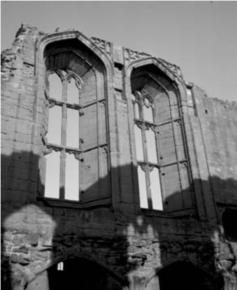
Figure 28. John of Gaunt's Hall, Kenilworth Castle, England, interior. The second-floor hall had huge windows looking out over a man-made lake. Deep embrasures would have created private spaces in the public hall. Because the floor is gone, one can see the change of masonry that marks the different levels. Photograph: Marilyn Stokstad.
