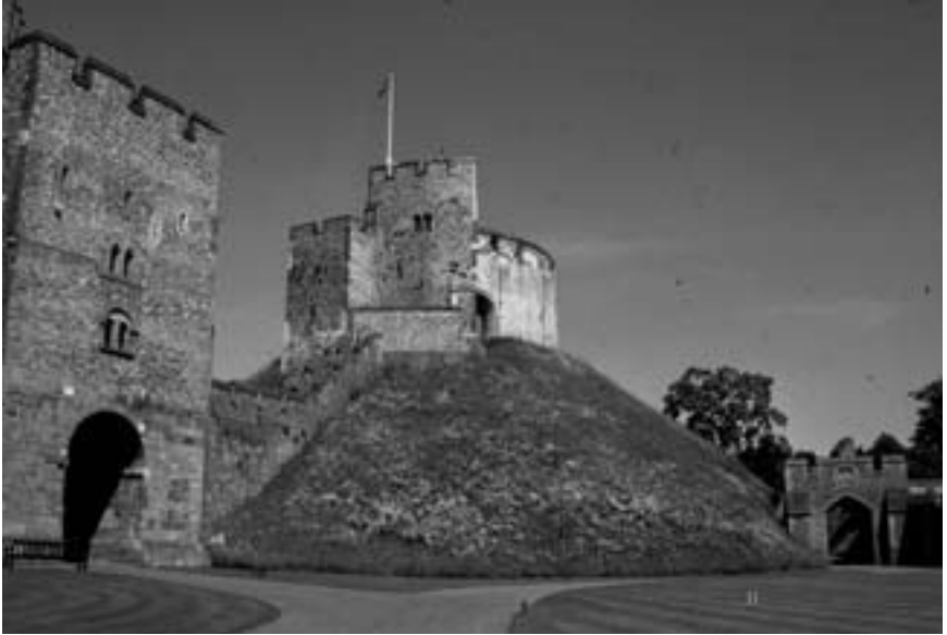
Figure 5. Norman motte, Arundel Castle, England. The motte at Arundel dates to c. 1088. William d'Abini (d. 1176) replaced the wooden structure on its top with the stone tower we see today. Like Windsor Castle, Arundel had a bailey on each side of the motte. Most of the castle buildings seen today were built in the 1890s. Photograph: Karen Leider.
