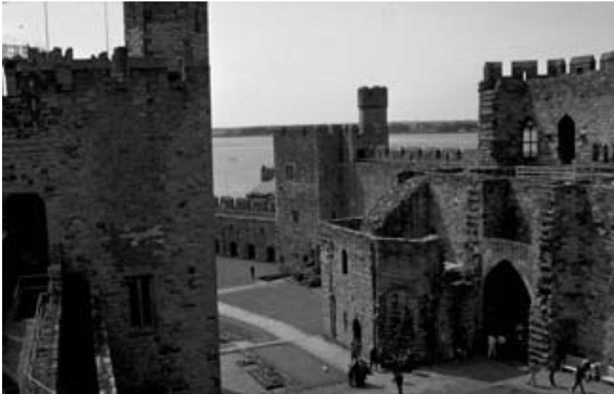
Figure 19. Gatehouse and lower court, Castle of Caernarfon, Wales. Built at the end of the thirteenth century, Caernarfon was the English king's governmental center in northern Wales. At the far right of the photograph is the King's Gate, the most complex gate built in medieval England and Wales. The lower courtyard contained the residence of the governor, a residence for the queen, and the great hall and the kitchens. The castle was accessible from the water and two watergates opened into this lower court. Photograph: Karen Leider.
