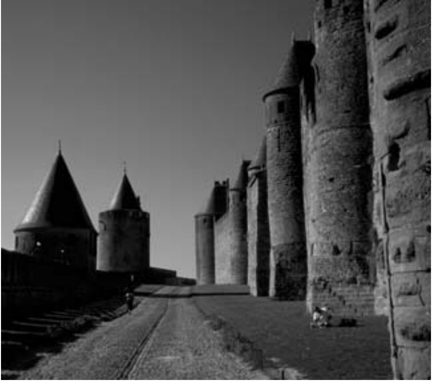
Figure 13. The walls and the lists, Carcassonne, France. The strongest castles and a few cities had double walls, a system perfected by the Byzantine builders of the walls of Constantinople. Archers on the high inner walls could shoot over the heads of men on the outer wall. The space between the walls, called the list, was used for exercise, training, and tournaments. Photograph: Karen Leider.
