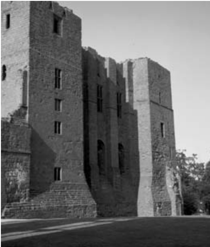
Figure 10. Great tower, Kenilworth Castle, England. The square tower with corner turrets continued to be built throughout the twelfth century. The large windows seen today at Kenilworth are the result of later modernization that turned the castle into a palatial residence. Photograph: Marilyn Stokstad.
