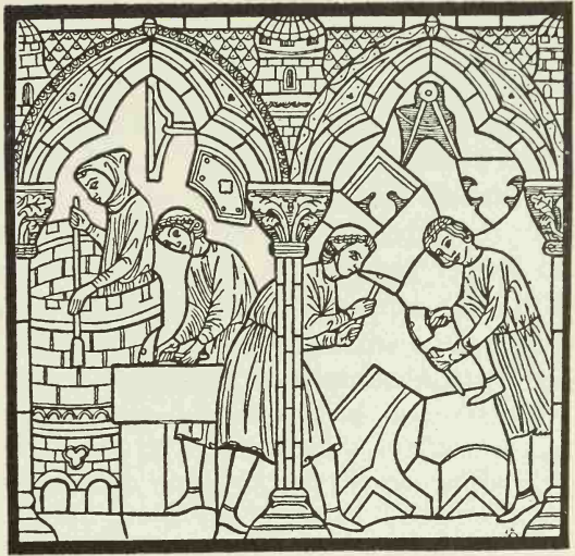
80 Carpenters and masons building Chartres Cathedral
