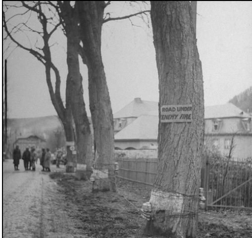
Trees wrapped with dynamite charges for use as a roadblock, near Malmedy, Belgium
