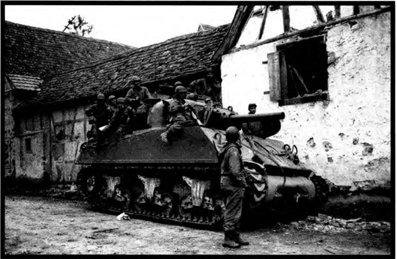
A modified M4 Sherman with a 105mm gun for close infantry support. A squad of American GIs ride on top.
