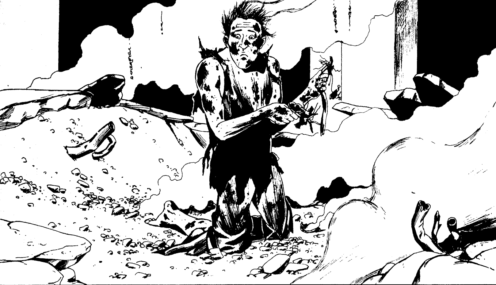
On-the-job training in demolition skill.
