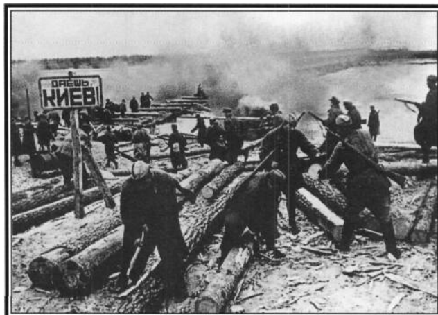
Below: Red Army engineers build a pontoon bridge across the Dnieper river on a bridgehead established to launch the offensive towards Kiev in October 1943. The sign exhorts them to greater efforts.
