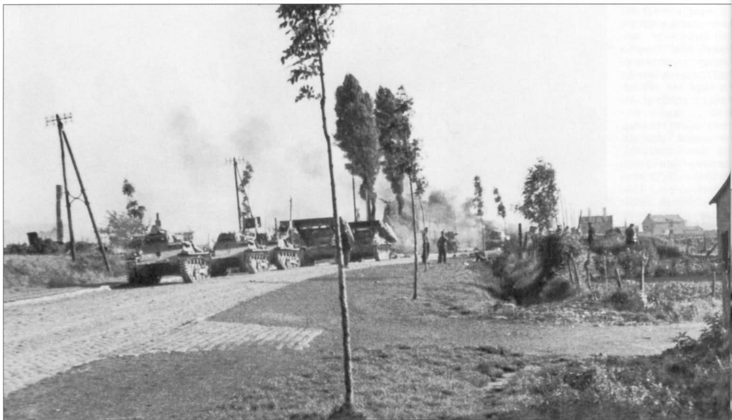
Each panzer-division's third company of its pioneer battalion was to be equipped with four Pz.Kpfw.IV bridgelayers for Fall Gelb. Due to shortages of equipment only half received the allotted numbers and the rest of the battalions were left to deal with the situation on their own. As shown here, Pioneer Bataillon 58 from 7.Panzer-Division equipped at least 2 standard Pz.Kpfw.II with bridges, although it is unclear if these were simply carried on blocks or if an actual launching mechanism was built. Leading the bridgelayers are three Pz.Kpfw.I Ausf.B.
