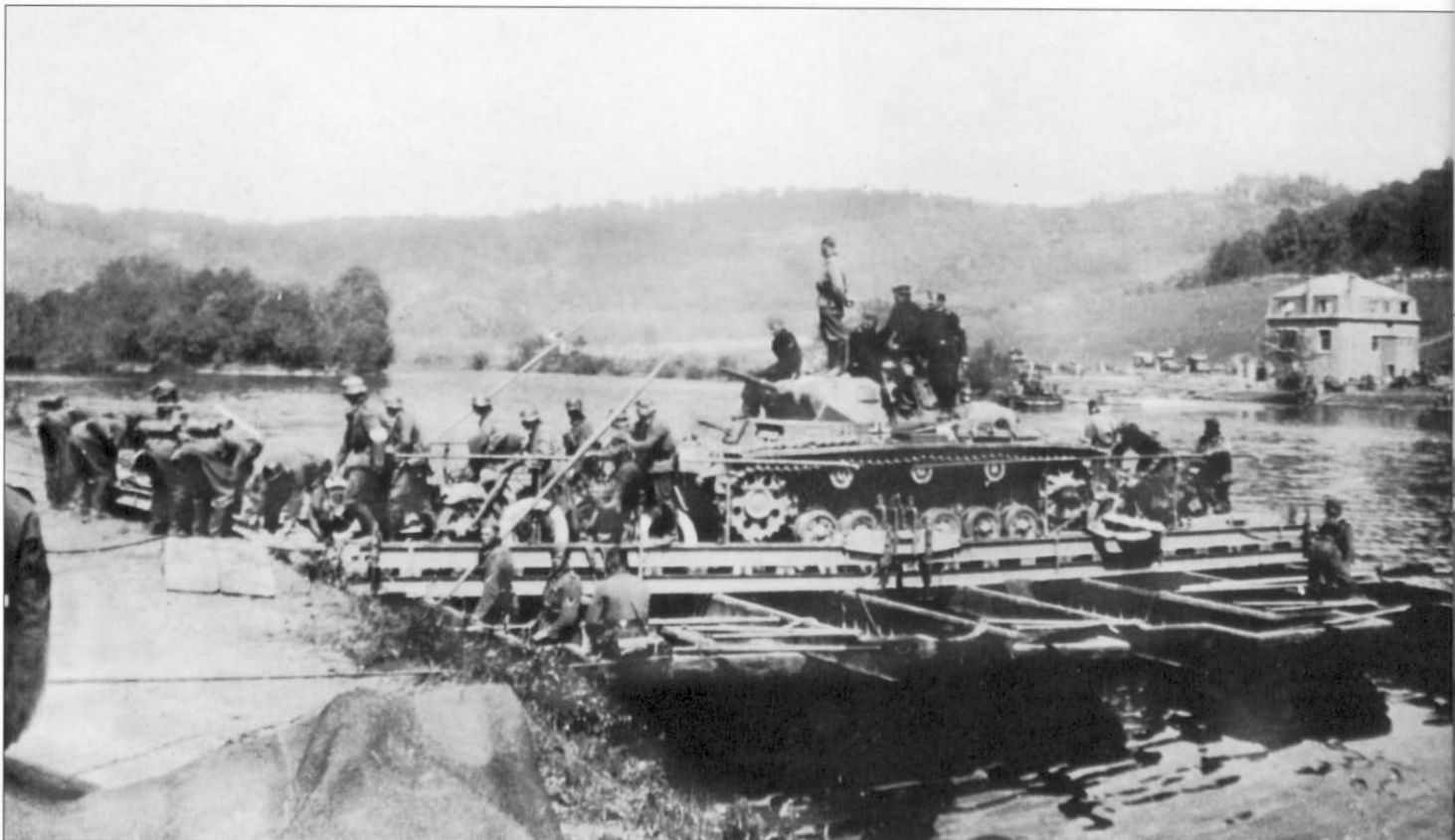
The Meuse was crossed by 5.Panzer-Division on May 13 to the south of Houx. Pontoon barges were used initially to ferry equipment across until the engineers could construct a pontoon bridge. Here, a Pz.Kpfw.III and group of motorcycles have just reached the west bank and are waiting for the offloading ramp to be emplaced. In the background can be seen many more vehicles and equipment waiting to cross.
