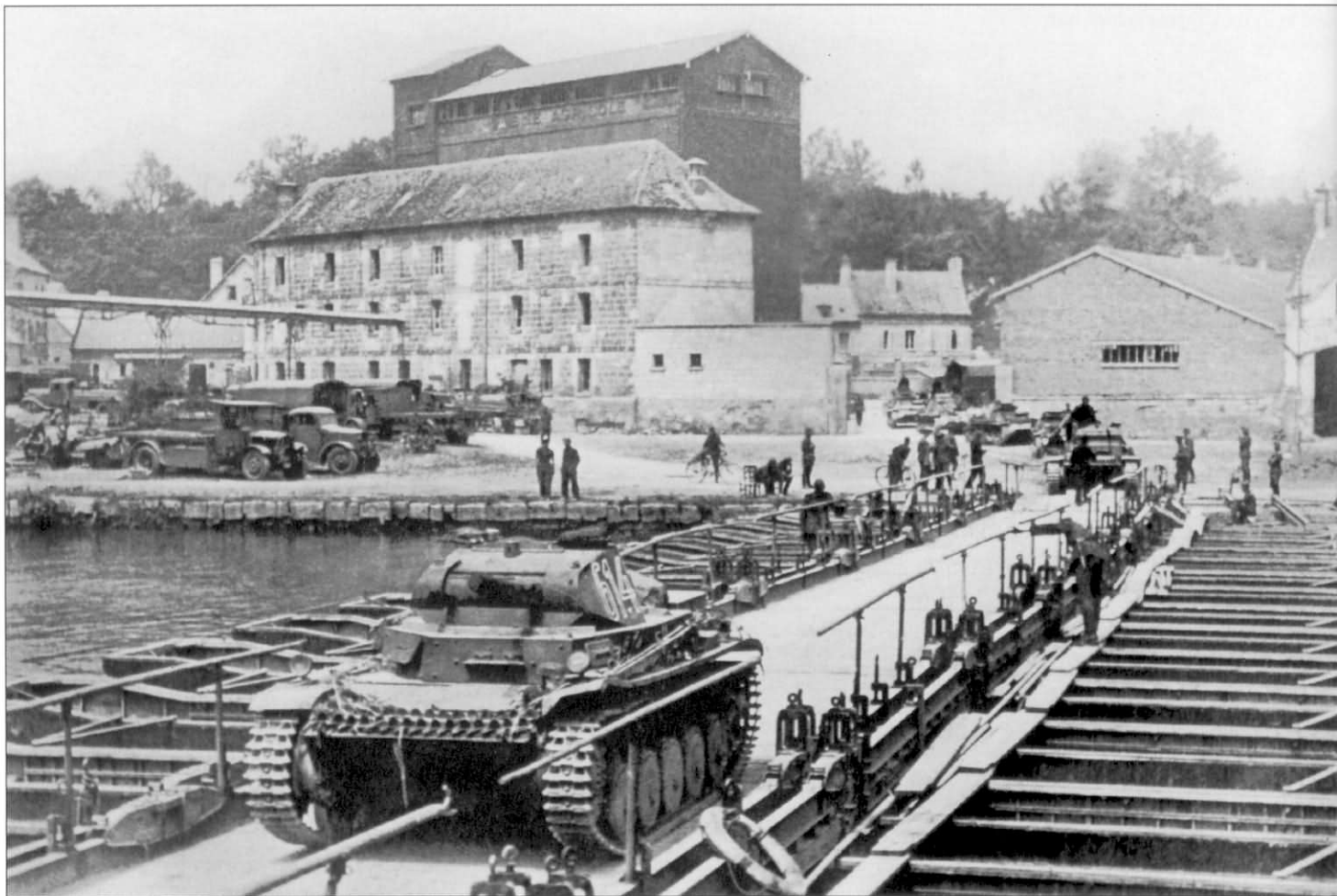
Pz.Kpfw.II "614" leads a column of Panzer Is, IIs and a Kl.Bef.Pz.Wg.I over a pontoon bridge across the Aisne River. In the background, the second tank is being directed onto the bridge after a considerable gap is left between the vehicles to insure that the capacity of the bridge is not exceeded. French trucks of all makes and models including civilian types are to the left.
