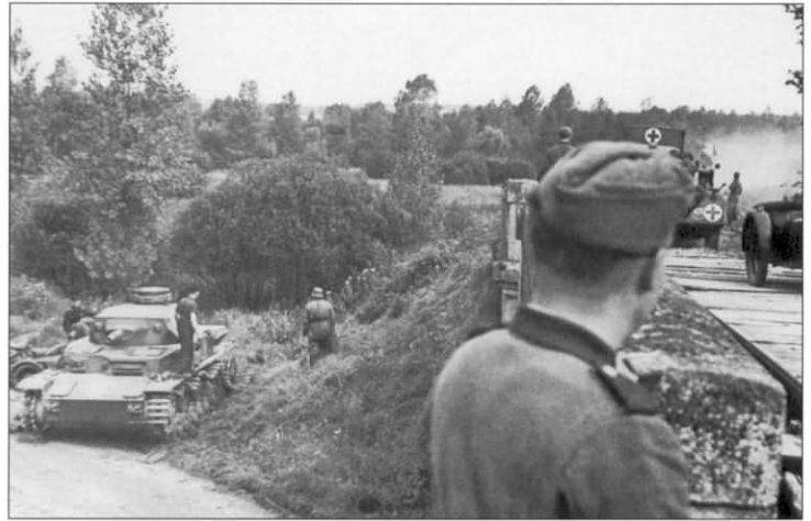
Finally, "321" has been dragged all the way to the bottom of the embankment so repairs can be made. A medical unit displaying prominent Red Cross symbols is moving across the bridge led by a motorcycle-sidecar combination.
