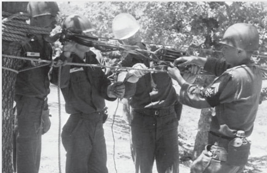
Combat engineers learned a great many skills during AIT at Fort Leonard Wood, Missouri, many of which proved useful to tunnel rats. Here trainees learn how to rig a block and tackle. (US Army)
