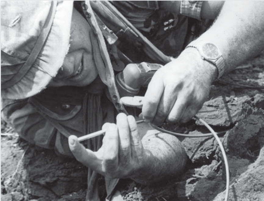
An M7 non-electric blasting cap is crimped to detcord using an M2 cap crimper. (1st Cavalry Division Museum)
