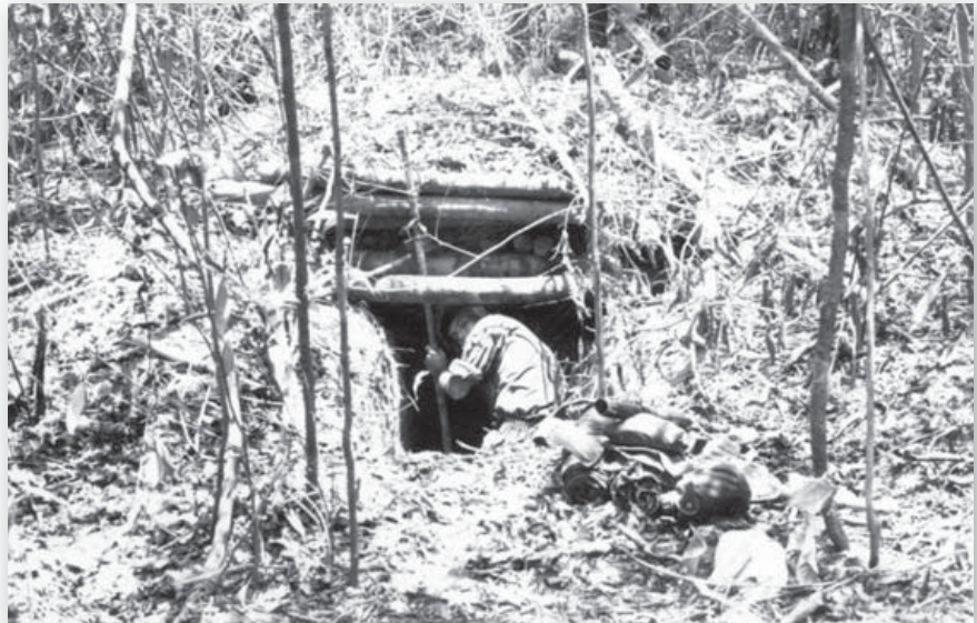
The camouflage has been stripped from this bunker. Several such bunkers were sometimes linked together by tunnels or simple shallow crawl trenches covered by camouflage. (Tom Laemlein/Armor Plate Press)
