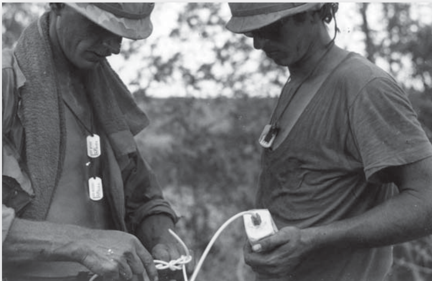
Engineers prepare 2½lb M5A1 C4 demolition charges and link them to detcord with half-hitch knots. The man to the right is wearing his helmet camouflage cover with the brown side out, which is unusual. (1st Cavalry Division Museum)
