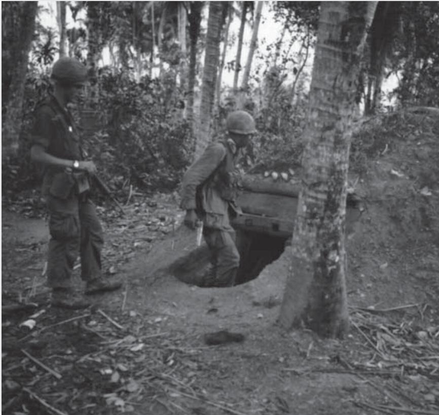
Bunkers such as these served as bomb shelters with roofs 4ft to 6ft thick made of crisscrossed logs and layers of earth. They had to be entered with care, because of the possibility of encountering booby traps. (Tom Laemlein/Armor Plate Press)
