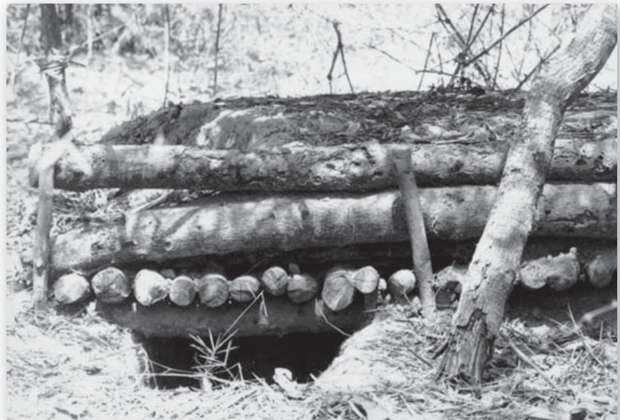
A crisscrossed log-constructed bunker. The tiny entrance was typical. This made it difficult for Americans to enter and complicated efforts to avoid or detect booby traps. (Tom Laemlein/Armor Plate Press)
