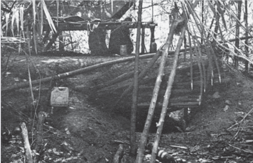
The entrance to a bomb shelter bunker in a trail rest camp. Note how heavily constructed the roof is, being made up of layers of logs and earth. There were always two entrances to relieve blast pressure. Bamboo benches and tables with a thatched roof shelter top the bunker.
