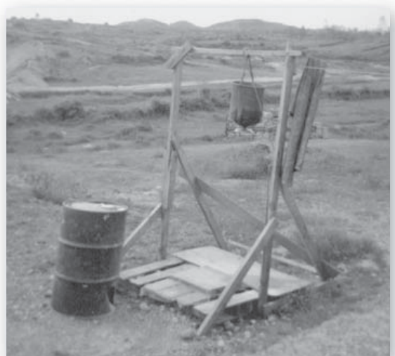
A crude field shower facility. The 3-gallon canvas shower bag was tuned on and off by turning the large shower head, which surprisingly built up more than adequate water pressure. A good shower could be had with just 4-5 gallons. (John Burford collection)
