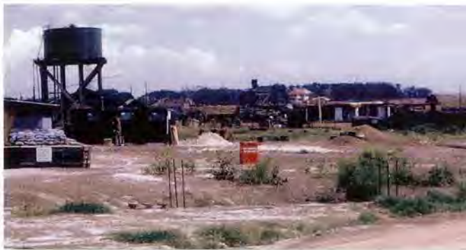
View of a typical larger base for a brigade or division on which many aviation units were stationed. Newly arrived officers would recommend that a machine gun be positioned atop water towers. That only attracted fire, making holes in the tower.
