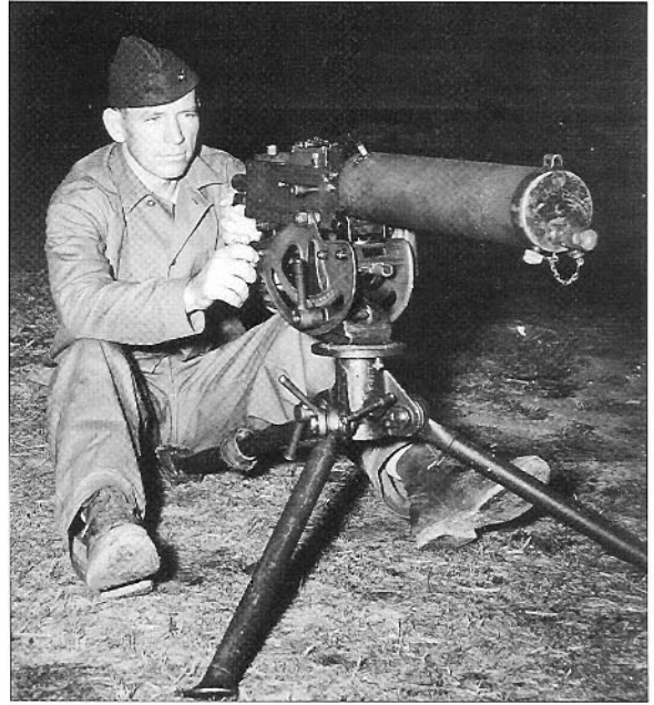
Machine gunners were trained on both the air-cooled M1919A4 light machine gun and the water-cooled M1917A1 heavy machine gun, pictured here. The brass water jacket end cap has been painted for camouflage and a blank adapter is fitted on the muzzle.
