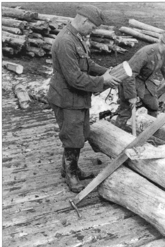
ABOVE The hard way to cut timber: the issue double-ended saw, here being used to cut timber for shoring up trenches and dugouts.
