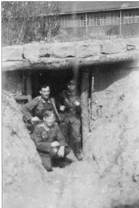
Another section position, well dug in with overhead cover, this time of thick concrete blocks.
