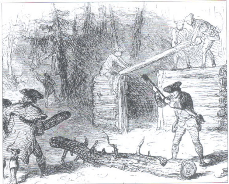
Building a Cabin. In fortified camps of a more permanent nature, Provincial and Regular soldiers were called upon to construct their own cabins or storage sheds. Many soldiers with a trade could earn extra pay for such work. (Dover Pictorial Archives)
