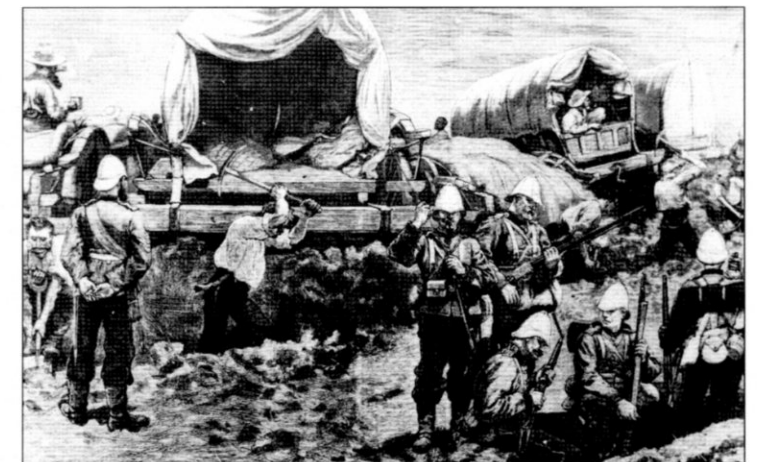
BELOW The 57th Regiment entrenching a wagon laager during the Eshowe relief expedition. According to the 1877 Field Exercise Manual, in 30 minutes one man could dig two paces (5ft) of shelter trench, 30in. wide and 18in. deep.
