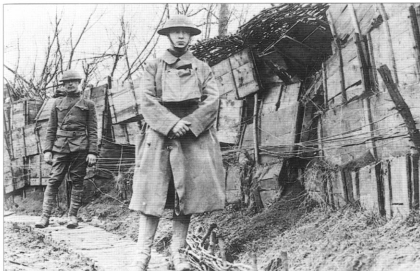
When the lines ran through particularly difficult terrain, such as swamps, instead of digging trenches the soldiers would construct barricades. This is an example of one of those barriers.
