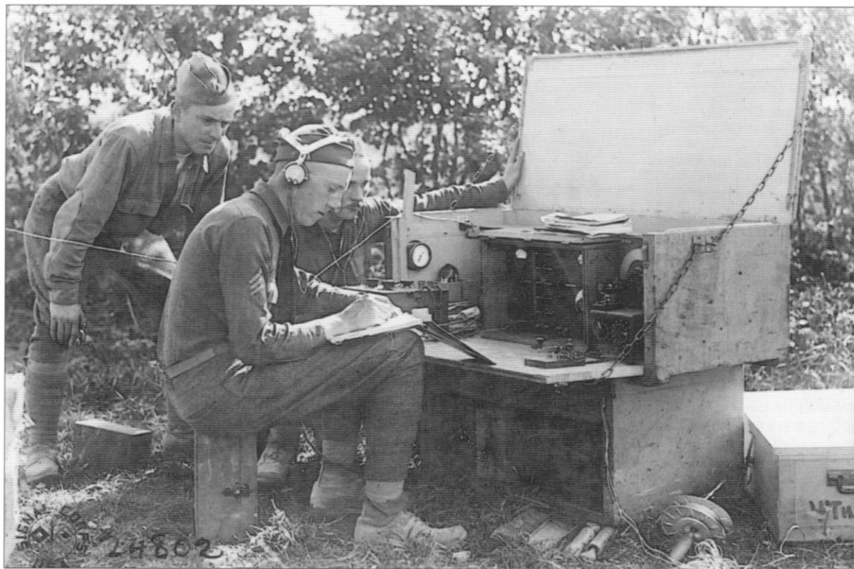
Sgt Edwin Wickliffe with his wireless, 80th Division HQ, Ippecourt, Meuse, September 16, 1918. Bulky and fragile, and therefore best left static, wireless communication was used to connect division to corps and army HQs. While not perfect, it was not susceptible to line breakage by artillery fire.
