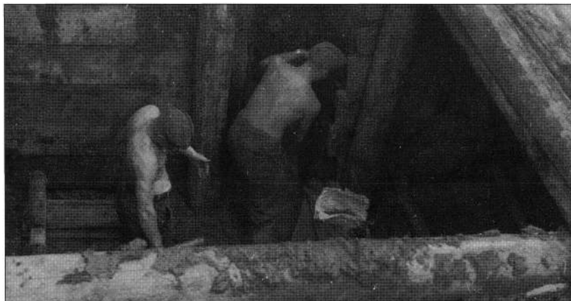
Troops constructing an underground shelter. Made of wood, these shelters were almost identical to the dugouts of World War I. They were used whenever there was time and timber available to construct them.
