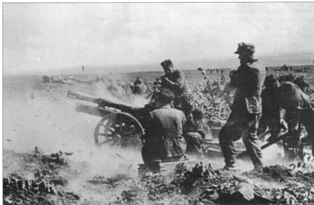
A 7.5cm Gebirgskanone in action. Note the compact size of this weapon, designed to be easily disassembled for transport by pack animals.
