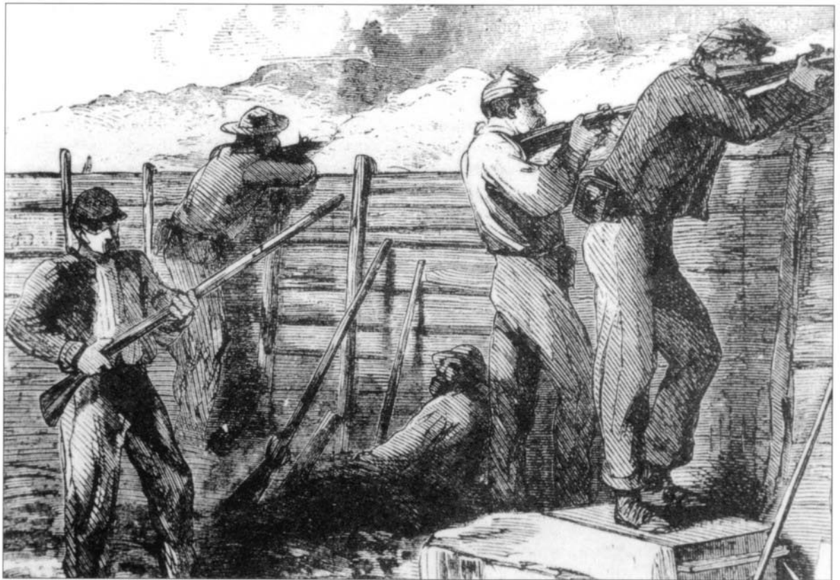
Once the siege had fully developed, trenches were built with wooden walls, firing steps, and slots in the earthworks for sharpshooters to use, as in this Harper's Weekly woodcut of Vicksburg.
