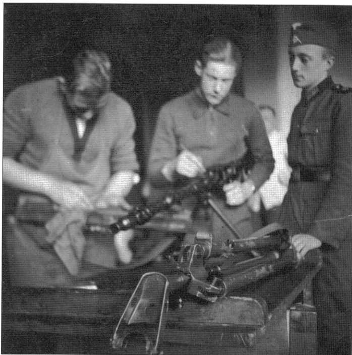
Two members of an MG team are seen cleaning the weapon under the supervision of the gun commander in 1938. The man on the left is cleaning a two-barrel spare barrel container. The man in the centre works on the breech mechanism of the gun, which has its bipod mounted in the mid-position. On the bench in the foreground is an anti-aircraft tripod, or Dreibein .
