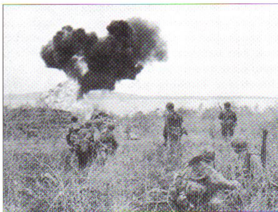
Saipan, June 17, 1944. Engineers flame the last of three bunkers. The two soldiers at right bottom are medics with the engineers. One wears two medical pouches with suspenders, the other carries a collapsible litter.
