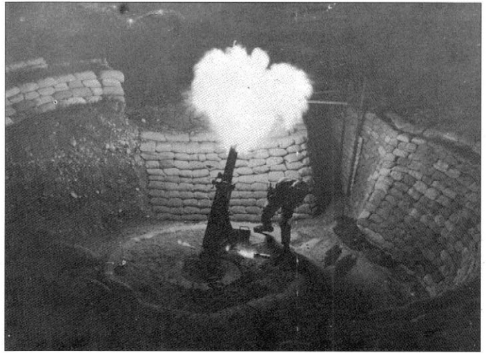
ABOVE The muzzle flash of a 4.2in. M30 mortar illuminates the interior of its pit. This particular example is larger than usually found. The exposed earth on the left side needs to be sandbagged before the wet season rains begin. Camp Thuong Duc, A-109, 1968.
