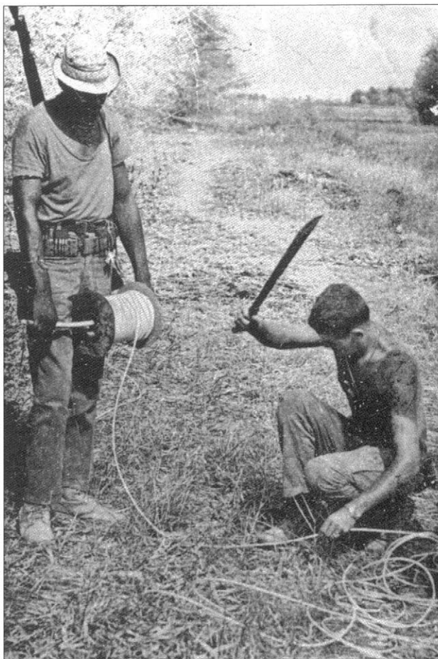
Two SF engineer NCOs cut a length of detonating cord to prepare demolition materials in order to clear trees hampering the approach to Camp Duc Hue's A-325 airfield. One man carries an M1 rifle with an M2 flash hider.
