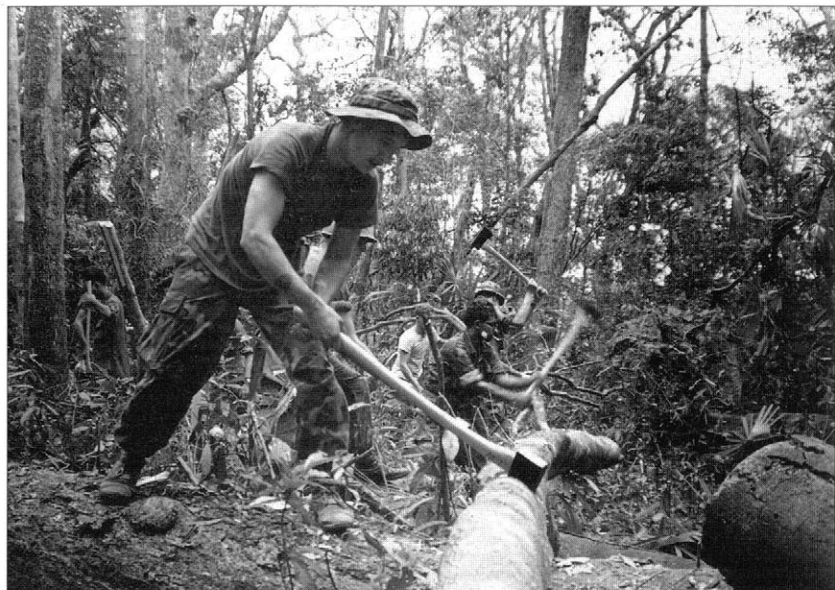
Groundwork included clearing trees and vegetation to allow helicopters to bring in engineer support and material to rapidly bring the fire support base into operation. The initial landing zones were levelled with hand tools. (DOD)
