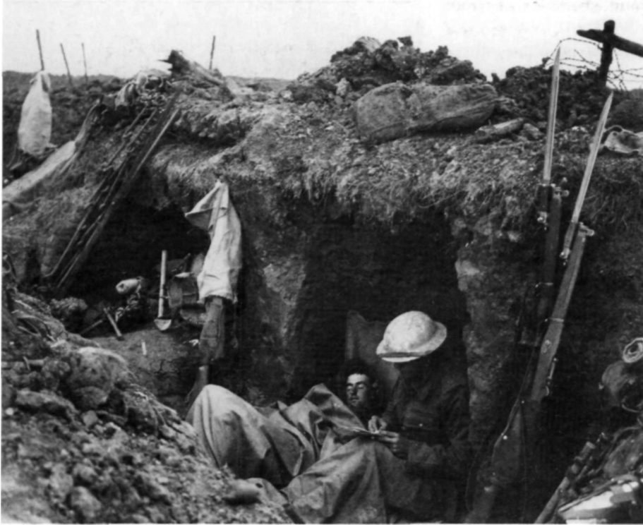
A good illustration of typical 'funk' holes'. Such hastily excavated dugouts provided the minimum of protection from weather and high explosive. Here, two men wrapped in ground sheets rest, surrounded by the litter of war. Two of the Enfield rifles visible have issue canvas covers over their actions, the two right-hand weapons being fitted with their 1907 sword bayonets. (Imperial War Museum)
