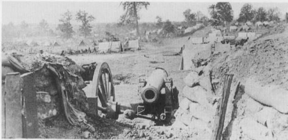
A 12-pounder Napoleon smoothbore in one of the Confederate redoubts protecting Atlanta in 1864. The Napoleon was the most widely used field gun of the war, more effective than rifled guns in the wooded and broken terrain that often dominated Civil War battlefields. Over 630 Napoleons were made in the Confederacy and 1,157 in the North. (US National Archives)
