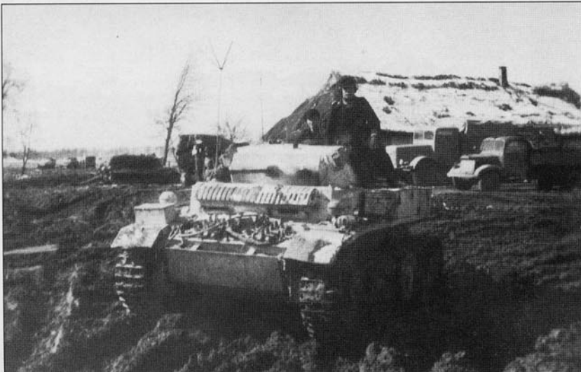
Two shots of a command version of the Pz.Kpfw.II Ausf.L 'Luchs' identified by the star antenna. In the above photo, the vehicle has become bogged down in the mud and the crew are working to free it. Even though it had a relatively high ground clearance, we can see that it has sunk down enough that the tracks can no longer move it. This is one of the original shipment of these vehicles received in the autumn of 1943 and has the spaced front armor plate and the spare idler rack on the front of the hull. The armor plate on the front of the 'Luchs' was only 30mm making it susceptible to small caliber Soviet anti-tank guns. The additional armor plate increased the protection to the equivalent of 50-60mm of armor plate.
