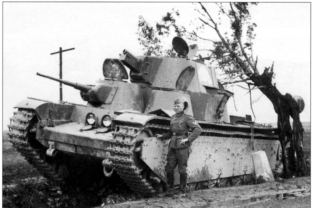
Another T-35 of 34th Tank Division that ended up in a ditch following a mechanical breakdown. Note the details visible on the deck. The Germans painted the white road markings for the safety of their drivers who were driving at night. They also removed the track, which was probably used to up-armor their tanks.
