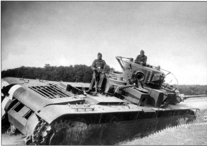
Another T-35 of 34th Tank Division that ended up in a ditch following a mechanical breakdown. Note the details visible on the deck. The Germans painted the white road markings for the safety of their drivers who were driving at night. They also removed the track, which was probably used to up-armor their tanks.
