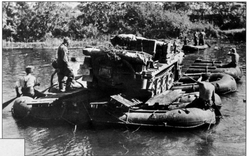
A Pz.Kpfw. IV Ausf. D in the so-called "U-bootpanzer" (Tauchpanzer) configuration, which permitted the tank to submerge in water up to 15 meters (16.5 yards) deep. These Tauchpanzer IVs were originally developed for the preparation of Operation "Sea Lion", the invasion of England, but were eventually used to cross the River Bug in June 1941 during Operation "Barbarossa". Note the frame around the turret front; this is the mounting frame for the waterproof fabric cover. The Tauchpanzers were mainly used by 18.Panzer-Division of Guderian's Panzergruppe 2.
