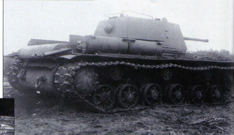
Another special purpose version of the KV-1 was the KV-12 chemical warfare tank. This had special cylinders mounted to the rear fenders. Although this could be used to dispense smoke, it was primarily intended to dispense chemical warfare gas. Chemical warfare never took place on the Eastern Front, so these were never produced in quantity. (R. Ismagilov)
