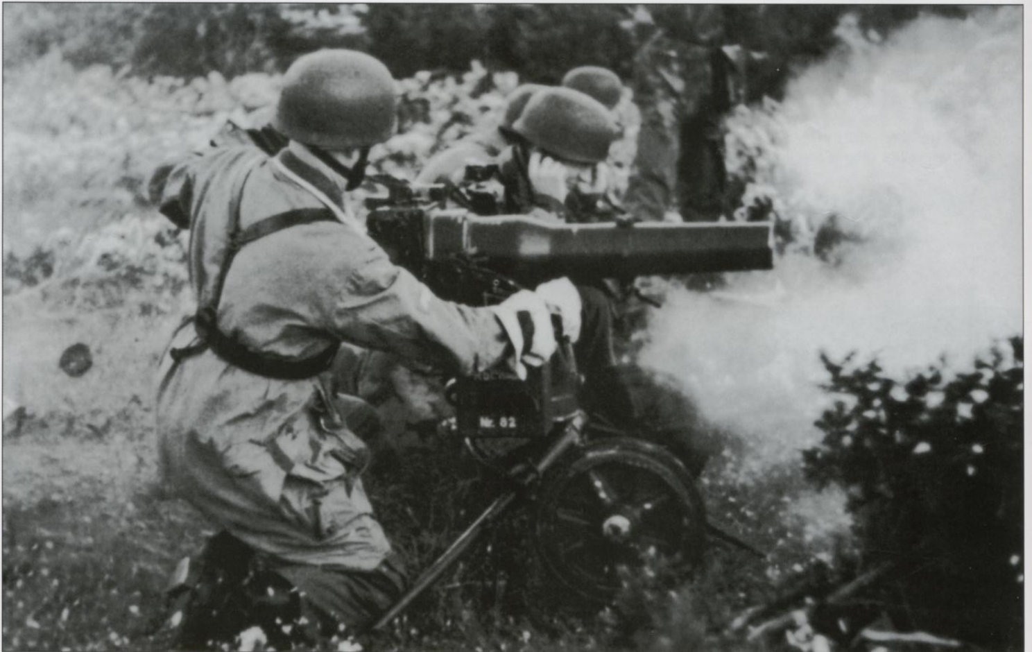
The 7.5cm Leichtgeschütz 40 recoilless rifle was the first gun of its type produced, being followed by the larger 10.5cm LG 40. The back blast was dangerous out to 50m during combat firing and crews were advised to plug their ears, as seen here, during firing as well. Only 450 of these guns were manufactured during the war.
