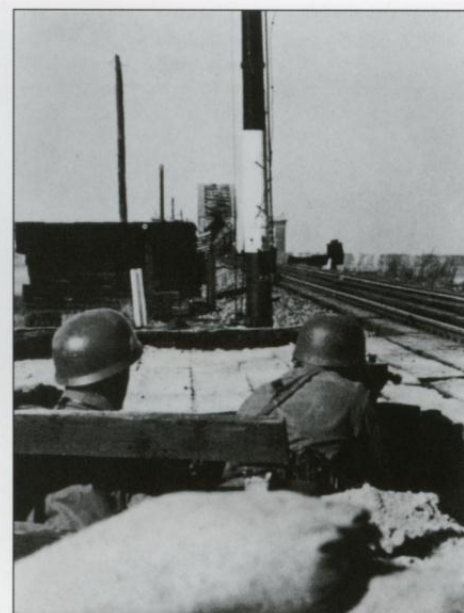
Paratroopers from II./FJR 1 man defensive positions on the Moerdijk rail bridge waiting for the Dutch to counter-attack. At 6:40 a.m. on the morning of 10 May, Leutnant Tietjen of 5./FJR 1 parachuted on to the bridge where he successfully neutralized the demolition charges paving the way for its capture. He was awarded the Knight's Cross on 24 May and promoted to Oberleutnant in October.
