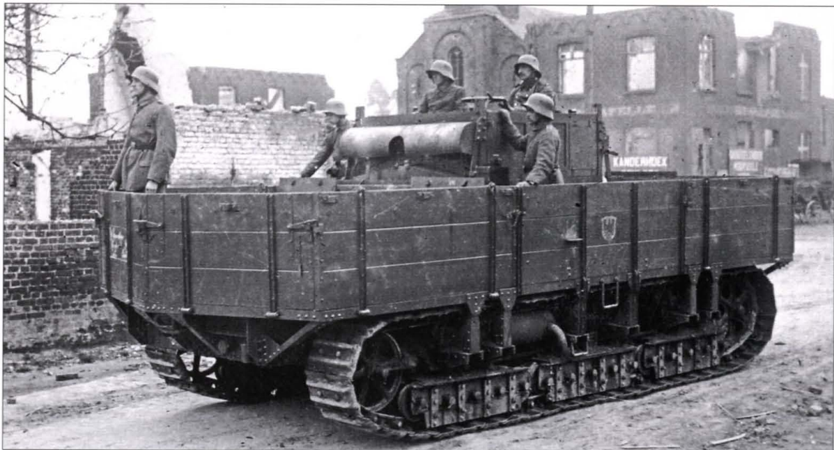
An A7V Gelandewagen moves through Ypres during 1918. In this view, the protective roof has been removed from over the driving compartment. (NARA)
