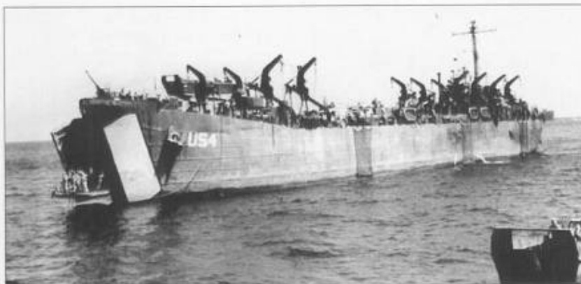
LST-4 approaches landing beaches in southern France. All but one of its six LCVPs have been launched. Three landing nets hang over the sides to allow troops to board landing craft. LST-4's hull number is preceded by the "US" required in the European-Mediterranean Theater.
