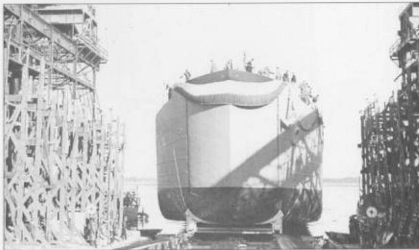
LST-357 sliding down the ways at Charleston Navy Yard, SC. Once launched it would require weeks of additional fitting before it was commissioned.
