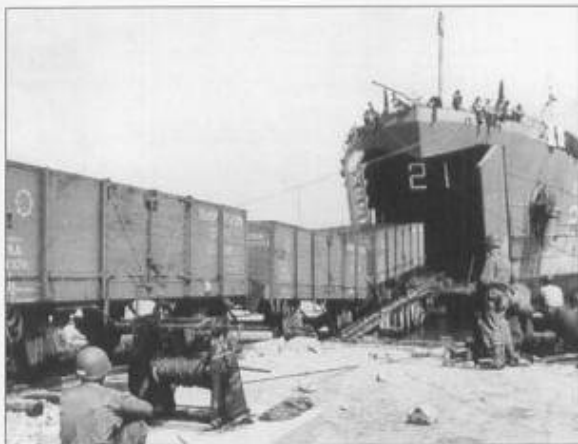
French-gauge railroad cars were delivered to Normandy by rolling them off special ramps on to rail extensions laid down the beach. Note the gondolas are marked with the US Army Corps of Transportation insignia.
