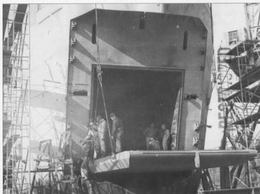
LST-157 under construction at Evansville, Indiana. Temporary cables support the ramp. The horizontal slots are for the geared door-closing ratchet and the upper vertical slots for the ramp chains. The heavy-duty door hinges can be seen along the sides. (Collection of the Evansville Museum of Arts, History and Science)
