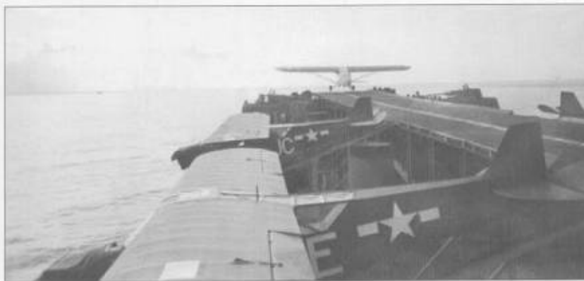
A Piper L-4 Grasshopper spotter aircraft launches from LST-906, one of six LSTs modified as "aircraft carriers" by Seabees (men of the US Naval Construction Force) in the Mediterranean. The flight decks were usually deck blue (dark blue) with a white or yellow center-strip. Others lacked the side storage racks.
