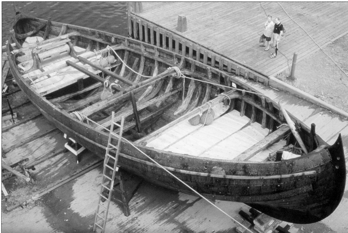
The Skuldelev 1 replica 'Ottar' under construction at the Museum shipyard, Roskilde. Note the cavernous cargo hold, the curving ribs and the sturdy crossbeams that brace her hull. (Photo Werner Karrasch, The Viking Ship Museum, Roskilde)
