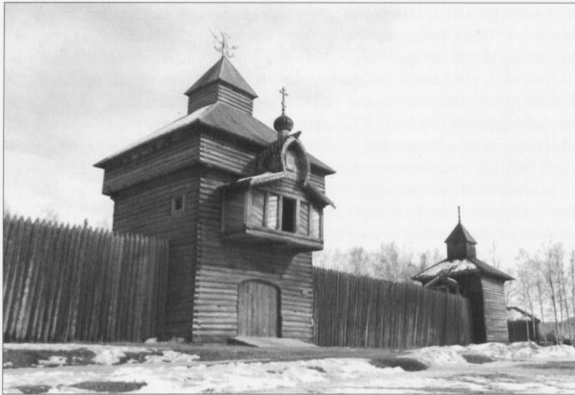
Gate tower of a mid 17th-century Russian wooden fortress, as reconstructed at the Taltsui Architectural & Ethnographical Museum. (Photo V.V.Tikhonov)
