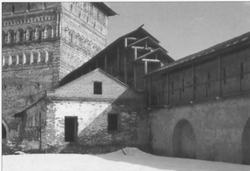
Great Tower and interior of the fortified wall of the 17th-century Spaso Preobrazhenski monastery, Suzdal. (Photo D.Nicolle)
