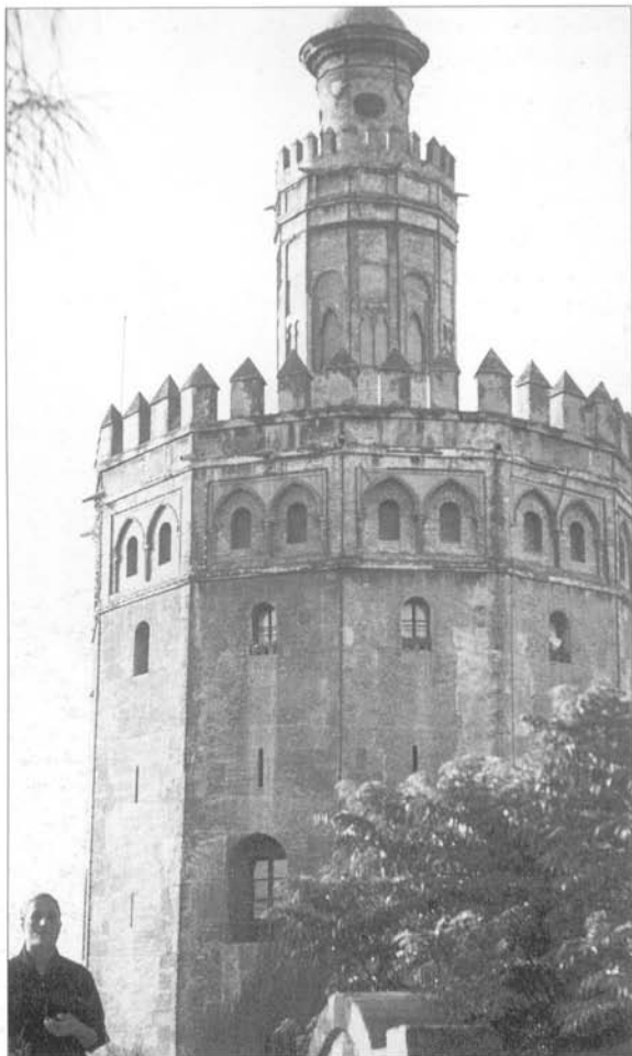
The Torre de Oro in Seville stands in the edge of the river Guadalquivir and was built in AD 1220. It was originally connected to the qasr main citadel by long ramparts, and served as a fortified outwork to ensure access to the river for water and communications. The twelve-sided main tower supports a smaller tower to which an additional cupola was added in the 18th century. (Author's photograph)
