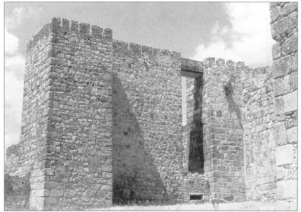
Trujillo castle was not one of the biggest frontier fortifications built by the Muwahhidun in the 12th and 13th centuries, but is one of the best preserved. Its barrana external towers are notable. This tower is now linked to the main wall by an iron bridge; the original would have been of wood. At the bottom of the gap between the barrana and the main wall is a small artillery emplacement added at a much later date. (Author's photograph)
