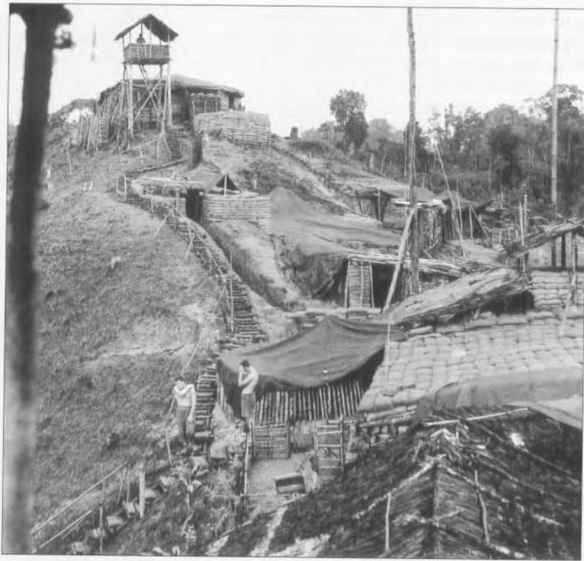
A typical border fort in Sarawak. It has an observation tower, bunkers made of logs and sandbags linked by communication trenches, and a stepped walkway up the hill – essential in the muddy conditions created by tropical rainfall – made of cannibalized ammunition boxes. Note the tall poles supporting radio aerials, and the vegetation cleared away to provide good fields of fire. (IWM FES 64/242/4)
