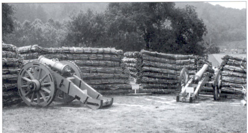
View of a reconstructed bastion at Fort Ligonier armed with, at left, an 8in howitzer and, at right, a 12pdr field piece. Pennsylvania, Delaware and North Carolina troops were among the garrison when the French attacked in the fall of 1758. (Fort Ligonier Museum)
