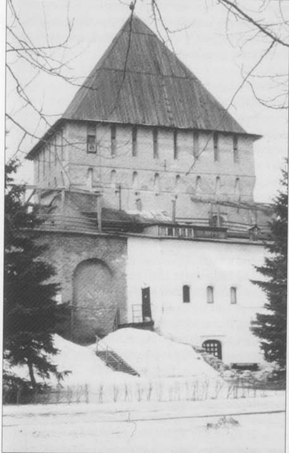
Tower Two of the Novgorod Kremlin. This particularly massive part of the brick fortifications was built in the 14th–15th C and is one of the earliest towers. (D.Nicolle photograph)
