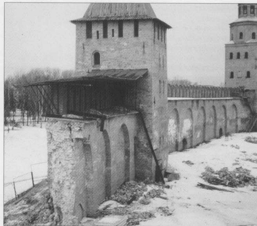
Tower Three of the Kremlin in Novgorod, seen from Tower Four. Tower Three is 15th C, and the broken wall between the towers can be seen to consist of two brick facings filled with a rubble core. (D.Nicolle photograph)
