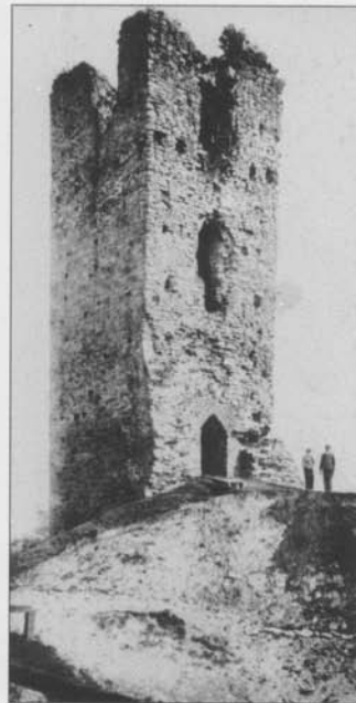
The fortified tower at Stolpye, built during the second half of the 13th or first half of the 14th century. Apart from a few largely symbolic stone gates in major cities, this type of isolated tower was the first form of stone fortification to be constructed in Russia. They appeared in the westernmost principalities, probably as a result of Central European influence, and would not be seen further east for many years.
