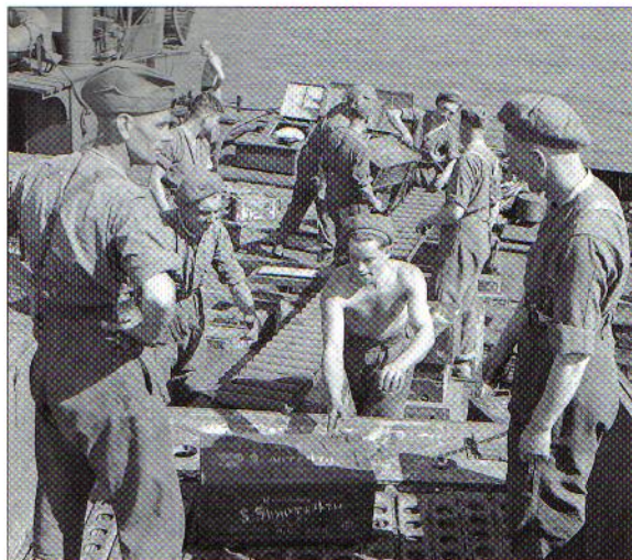
Normandy, June 1944: shirt-sleeved pioneers, wearing a mixture of FS and GS caps, manhandle cased 5.5in rounds over a conveyor on 'Mullberry B', the British prefabricated harbour established off Arromanches. The build-up of forces in France required a huge input of every kind of equipment and stores. By the end of August 60 per cent of the matériel in Normandy had come ashore straight across the beaches via LSTs and amphibious DUKWs, with another 20 per cent through the two Mulberry harbours and an equal amount through Cherbourg and smaller ports. (IWM BU703)
