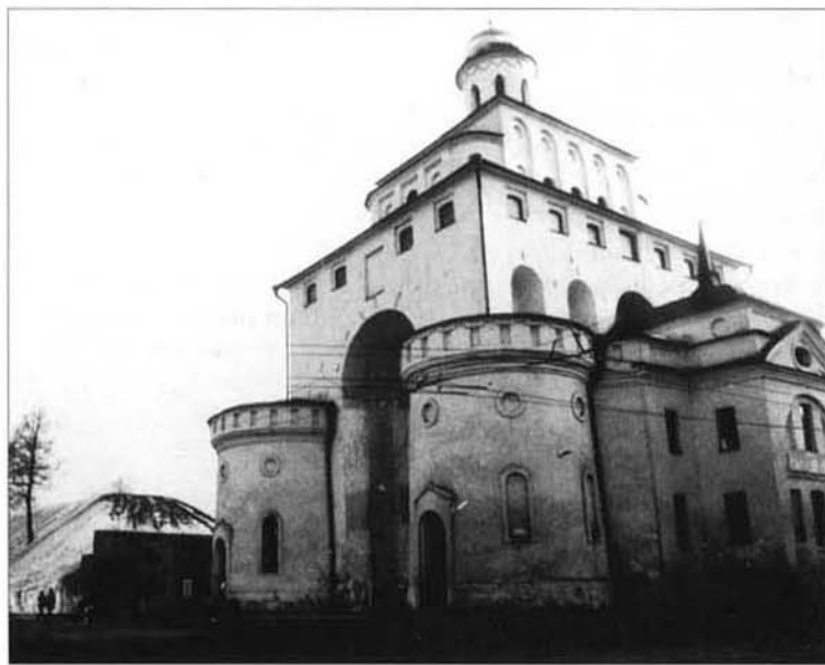
The Golden Gate of Vladimir today; it was originally built in 1164 without the circular corner buttresses. (Author's photograph)
