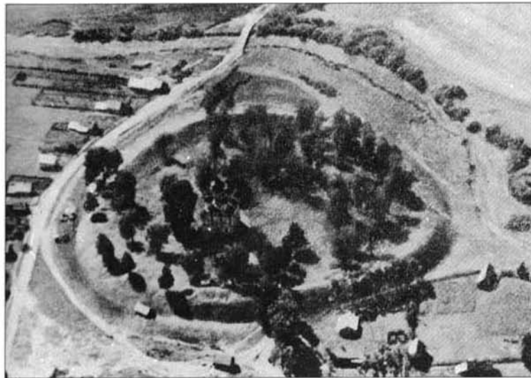
Aerial view of the site of the 12th century fortified settlement of Mikulin. (APN photo)
