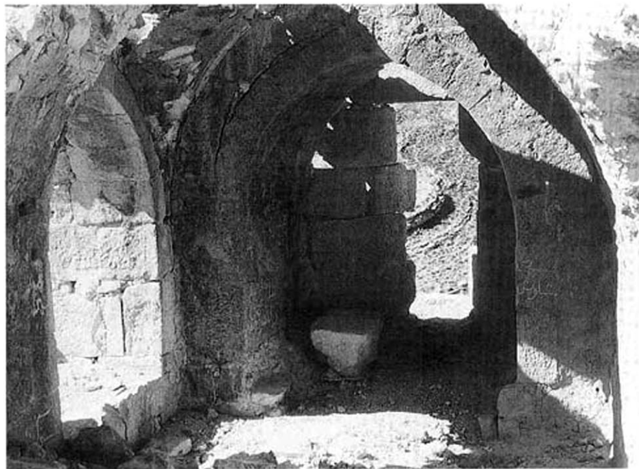
Shawbak in southern Jordan is often called a Crusader castle, but the existing structure was rebuilt and greatly enlarged by the Mamluks. This picture shows several firing or observation positions within its massive wall. (Author's photograph)
