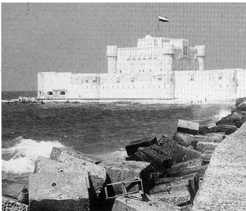
On a different scale to other mamluk fortifications is Sultan Qait-bay's castle overlooking Alexandria harbour. It was completed, with gunpowder artillery in mind, in 1479, and consists of a large inner citadel surrounded by a strong but lower outer wall. (Author's photo)
