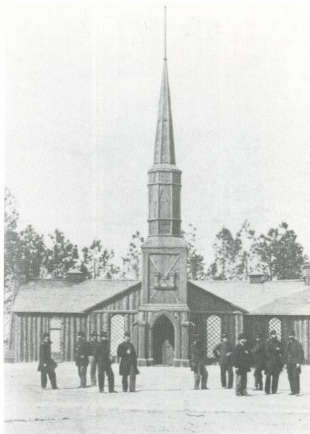
The Corps of Engineers of the Army of the Potomac built this chapel behind the lines at Petersburg, 1864. Note how they have worked the Corps insignia out of logs over the door. Corps officers and enlisted men stand in front of their work. (Library of Congress)
