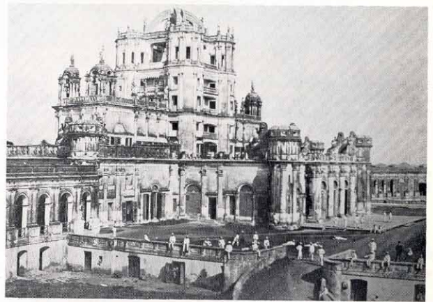
24. La Martinière, Lucknow, built in the Italian style in the late 18th century by a French general then employed by the ruler. At the time of the Mutiny it was used as a boys' school. It was fortified by the mutineers during Sir Colin Campbell's attack on the city.
