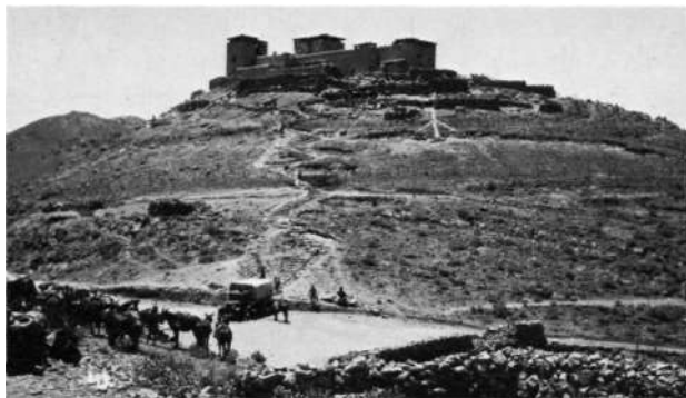
Thal fort overlooking the Tochi River at the point where the Bannu-Razmak road crossed the river. It was normally garrisoned by a company. The watch-towers have been roofed in to keep the sun off the sentries. (Photographed by R. B. Holmes of Peshawar)
