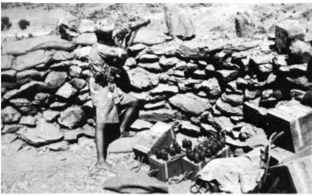
A post on the perimeter. The upright headstones on the tops of the wall were to break up its outline and prevent the head of the sentry from being silhouetted. The post had been plentifully supplied with grenades
