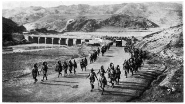
The Bannu-Razmak road. 'D' Company on the line of march, May 1940. (Photographed by R. B. Holmes of Peshawar)
