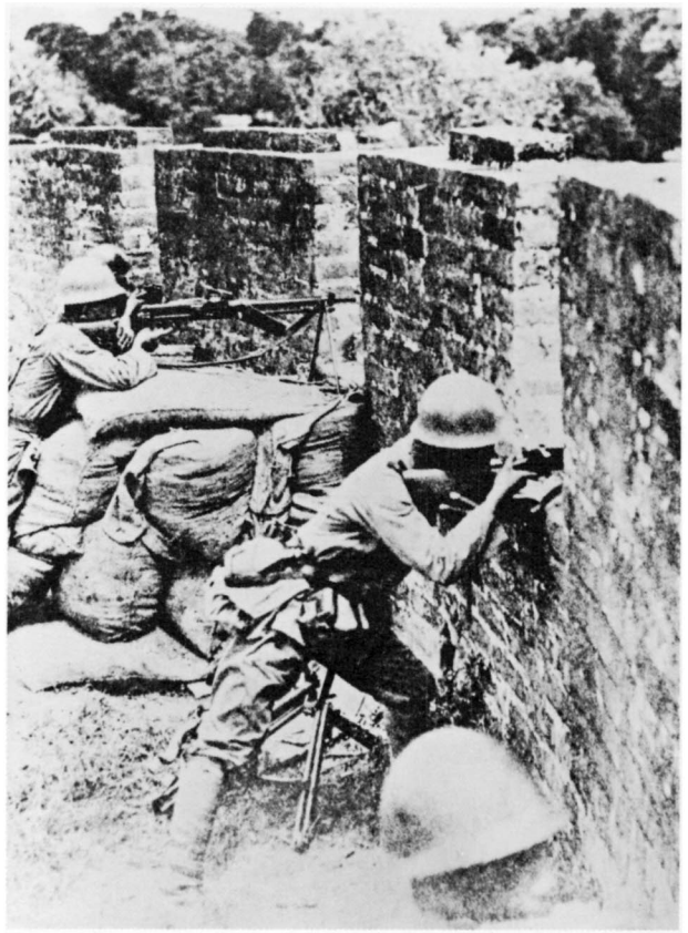
The soldier in the background is firing the standard Japanese light machine-gun at the outset of the war, the 1922, Model 11, gas-operated air-cooled gun of 6.5 mm. calibre. It only operated correctly with reduced-charge rifle cartridges, six clips of five rounds each being fed into the open hopper on the left side of the breech. (Imperial War Museum)
