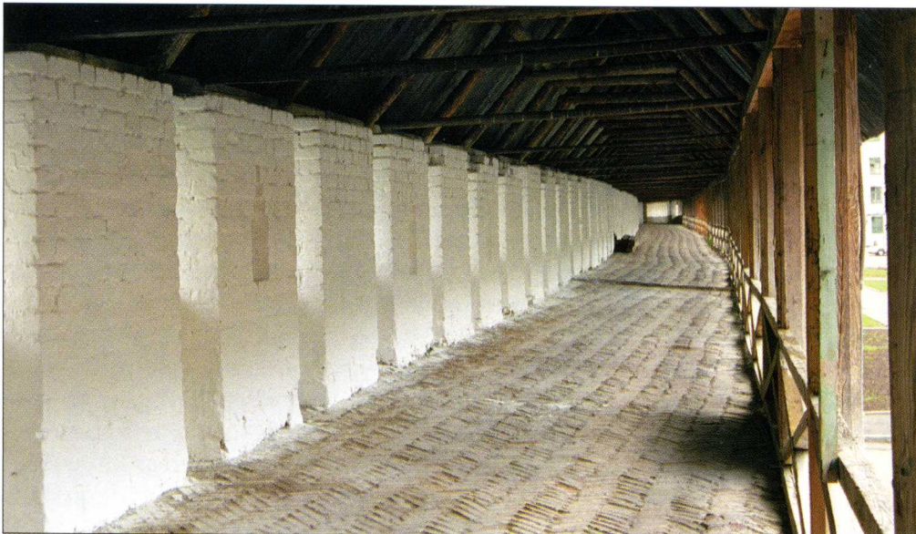
The gallery behind the parapet (wall-walk) in the Kazan Kremlin. Historically, the boevoy hod (wall-walk) in all fortresses had wooden roofs. The roofs haven't survived and now can only be seen where they have been reconstructed, as here.
