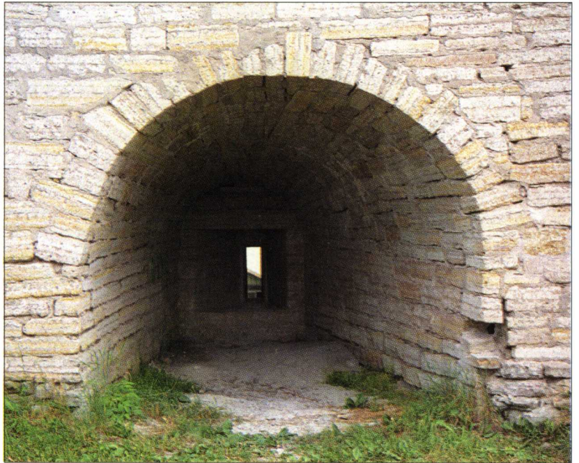
Interior view of a chamber ( pechura ) in the bottom tier of the wall ( podoshvenny boy ) of the fortress of Ladoga.
