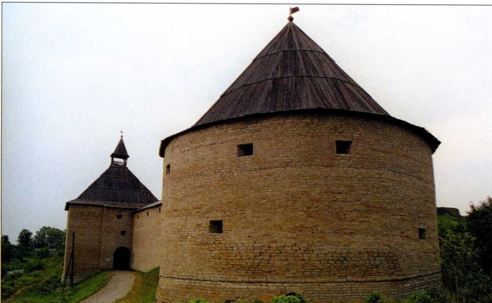
A general view of Ladoga Fortress. It had five towers, some of them round, some rectangular.
