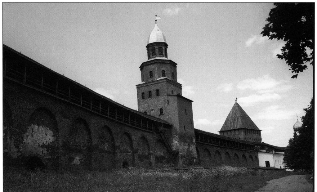
An inside view of the wall surrounding the kremlin of Novgorod the Great. Arches inside walls became very common in the 15th–16th centuries. Some of the arches had chambers ( pechuras ) where cannon were emplaced.
