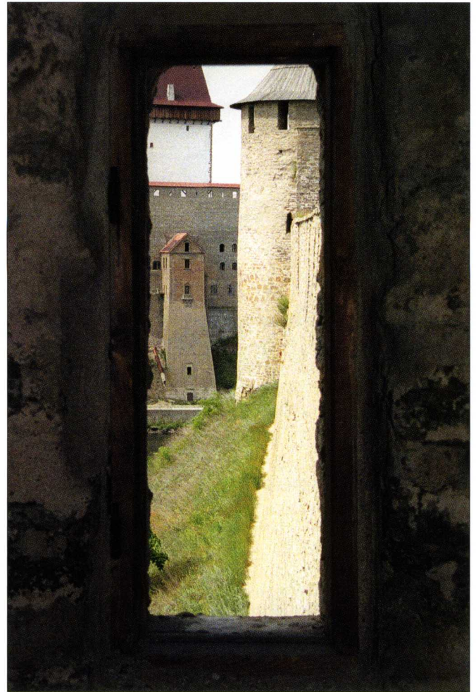
View through a loophole in the Shirokaya (broad) Tower of Ivangorod. Note how well the entire space at the foot of the wall can be covered by fire.
