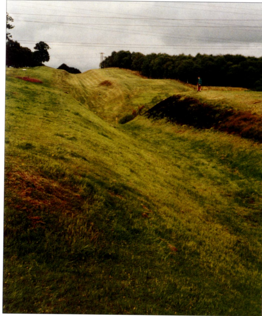
The Antonine Wall ditch west of Rough Castle. On the left of the ditch is a low mound, all that remains of the turf rampart that once stood at a height of 2.75m. This was topped with a 1.85m-wide wooden duckboard walkway protected by a split-timber or wattlework parapet 1.5m high. (Author's collection)
