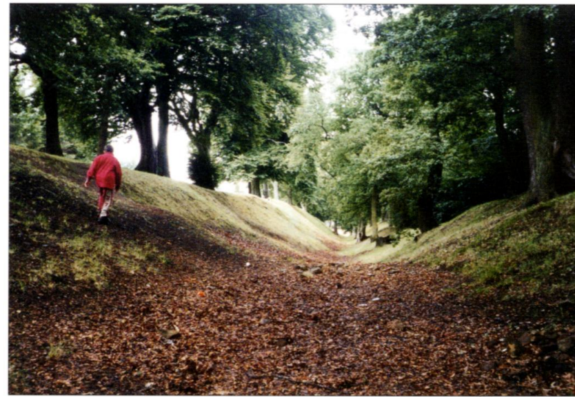
The Antonine Wall ditch at Watling Lodge, looking west. Here it presents the visitor with a formidable barrier, preserving almost its original dimensions of 12.2m in breadth and 4.5m in depth. Like most military ditches, it is V-shaped in profile, the scarp and counter-scarp sloping up at an angle of 30 degrees to the vertical. (Author's collection)
