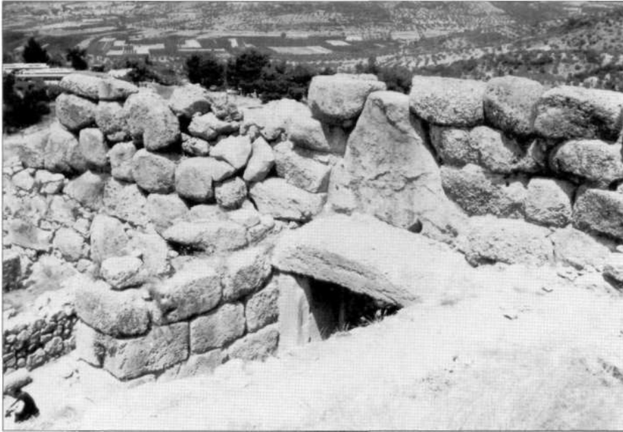
LEFT The inner facade of the Lion Gate, showing the conglomerate lintel estimated to weigh in excess of 20 tonnes. Above the lintel block, so as to reduce the load resting upon it, the wall was corbelled to leave a relieving triangle, in which is set the famous limestone relief of lions (more properly, lionesses) flanking a column, the back of which is seen here. (Author's collection)
