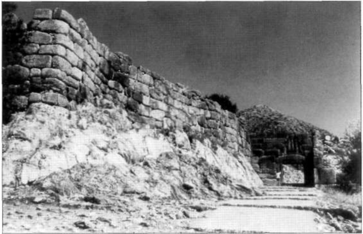
The Lion Gate at Mycenae, made famous by the heraldically opposed felines above it, is in fact carefully arranged so that any potential attacker can be attacked from the salient of the fortification walls that flanks the left-hand (north-east) side of the approach route. The situation was made even more lethal for the attackers by the presence of the rectangular bastion immediately to the right (south-west) of the entrance passage. (Author's collection)
