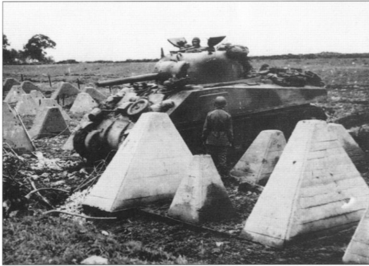
An American Sherman tank follows the path blasted by US Army Engineers during the fighting around Aachen in September 1944. The Americans tended to attack road blocks rather than sections of dragon's teeth because destroying the teeth was dangerous and time consuming. (Imperial War Museum)
