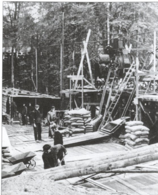
The construction of the West Wall employed the majority of the country's concrete mixers. Cement, sand and gravel were loaded into hoppers at the bottom and lifted up to the mixers which could then pour the mixture in the desired place. October 1938. (Bundesarchiv)
