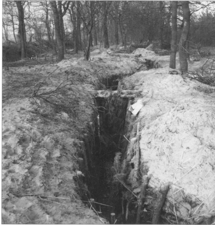
The defences to the north of Aachen (with the exception of those around Cleve) were less well developed than those to the south. Often they consisted of barbed wire entanglements, or, as here, revetted trenches. When the West Wall was originally built the border with Belgium and the Netherlands was not considered a priority. (Canadian National Archives)
