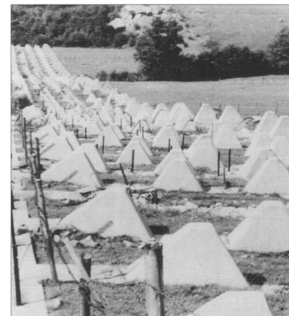
In front of the main defences, the Germans constructed miles of concrete anti-tank obstacles, or dragon's teeth. The enemy would advance from the left and would be confronted by rows of increasingly large concrete teeth. To hamper the infantry, iron stakes were strung with barbed wire and were positioned along the length of the line. (Public Record Office)
