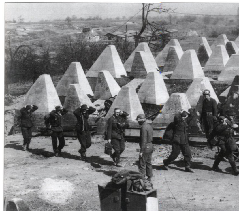
American military policeman process German POWs as they pass through a section of dragon's teeth. The pristine looking teeth appear to be of the larger type 1939 pattern which were built to counter the development of bigger more powerful tanks. The teeth to the right appear to be originals painted green to merge in with the landscape. (Imperial War Museum)
