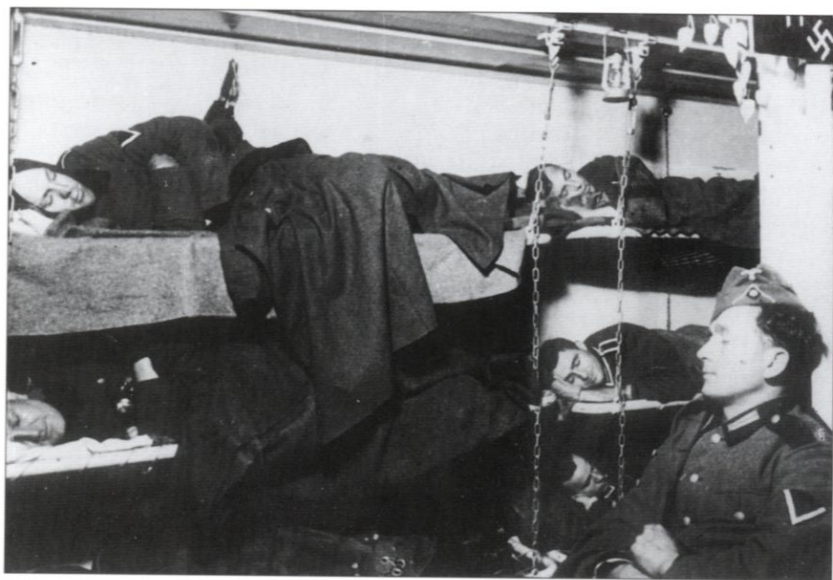
ABOVE The crew of the West Wall bunkers were afforded few luxuries, but most shelters were fitted with beds. The three tiered bunk beds were suspended on one side by chains fixed to the ceiling and on the other by hinges so that they could be folded against the wall when not in use. The steel framework was fitted with a wire mesh over which was stretched a sailcloth. A mattress and pillow were also provided. (Author's collection)
