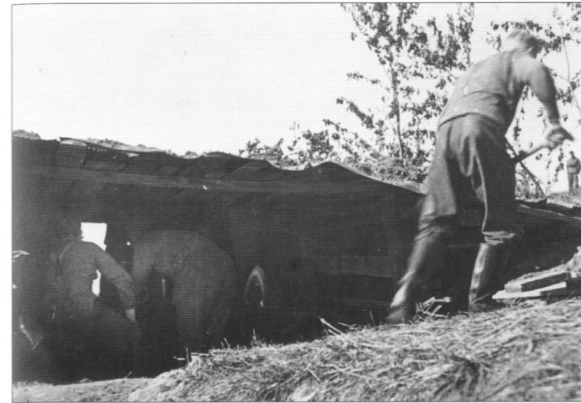
The early defences of the West Wall were very primitive. Here an anti-tank shelter near Pirmasens has been prefabricated out of wood which is being covered in spoil for added protection. Just visible in the gloom is the outline of the anti-tank gun. (Imperial War Museum)
