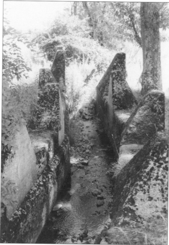
Where no natural obstacle barred the passage of tanks, engineers constructed rows of concrete anti-tank obstacles, or dragon's teeth. Inevitably, it was necessary to include breaks for roads, tracks and in this case a small stream. This obstacle is still visible and is located near the village of Lammersdorf. (Author's collection)
