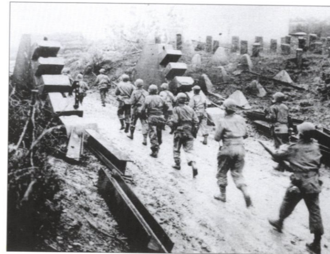
Men of the 39th Infantry Regiment (9th Infantry Division) pass through the Siegfried Line near Roetgen. In the immediate foreground are iron girders that were placed in the recesses of the trägersperre to block the road. To the sides are dragon's teeth and improvised anti-tank obstacles which are simply wooden posts rammed into the ground. (US National Archives)
