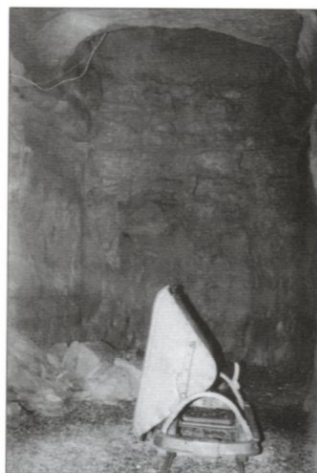
The tunnel system of the Gerstfeldhöhe was designed to have two levels – an upper or fighting level and lower or storage/sleeping level. To link the two a 68 metre high lift shaft was to be constructed. The hole was bored, but the lift was never completed. (Author's collection)
