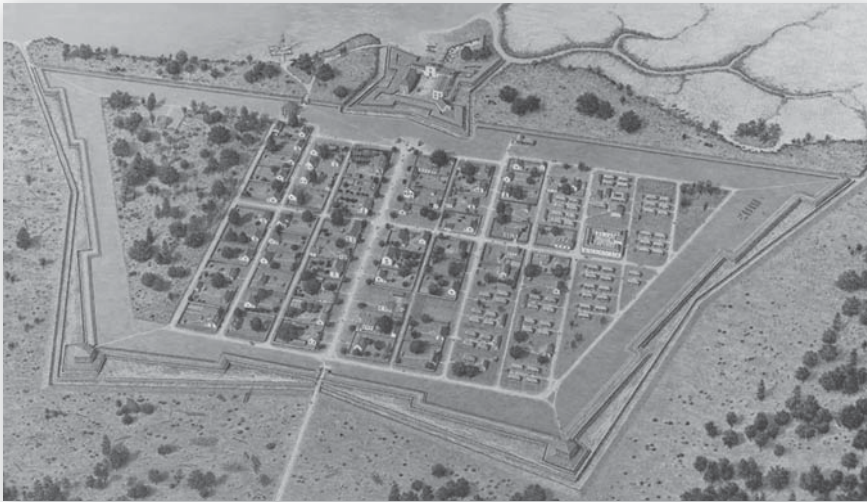
Frederica, Georgia, 1736–48. The fortress settlement of Frederica was established three years after the foundation of the colony of Georgia to secure the contested southern frontier with the Spanish in Florida. The town was protected by curtain walls made of earth and cedar posts that were about 10ft (3.04m) high, the landward side being surrounded by a moat. The adjoining Fort Frederica (top) acted as its citadel, featuring three bastions and a projecting spur battery of 18-pdr guns to engage enemy ships. There was also a fortified military barracks in the town (right of picture). (Painting by L. Kenneth Townsend. Fort Frederica National Monument, US National Park Service)
