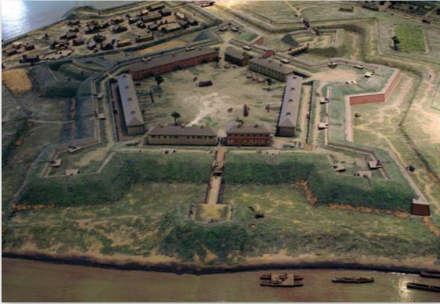
Fort Pitt, 1761–72. This very large fort consisted of an earth-and-timber pentagon with five large bastions. The bastions and curtain walls on the landward side were faced with bricks. Outside were ditches, glacis, a ravelin, and a small village also protected by earthworks. (Fort Pitt Museum, Pittsburgh)
