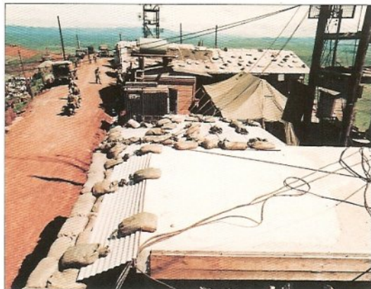
A complex array of antennae and other communications equipment at an elevated hilltop position, 4th Infantry Division, June 5, 1969. Once again we find that the vital electronic part of a firebase's function was necessarily the least well protected from enemy fire. By the same token the sparse scattering of sandbags over the corrugated steel roofing was designed to hold it down in high winds rather than to afford protection against mortar bombs. (US National Archives)
