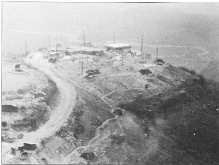
Hilltop retransmission site at FSB T-bone (Thua Thien province) in 1971. It commanded an excellent direct view of Hue, and hence excellent conditions for radio transmissions. Note the inner "keep" for all the clever technical stuff is at the summit (with an MPQ-4 counter-mortar radar just to the left), while the perimeter defense bunkers are scattered around the slopes below. (US National Archives)
