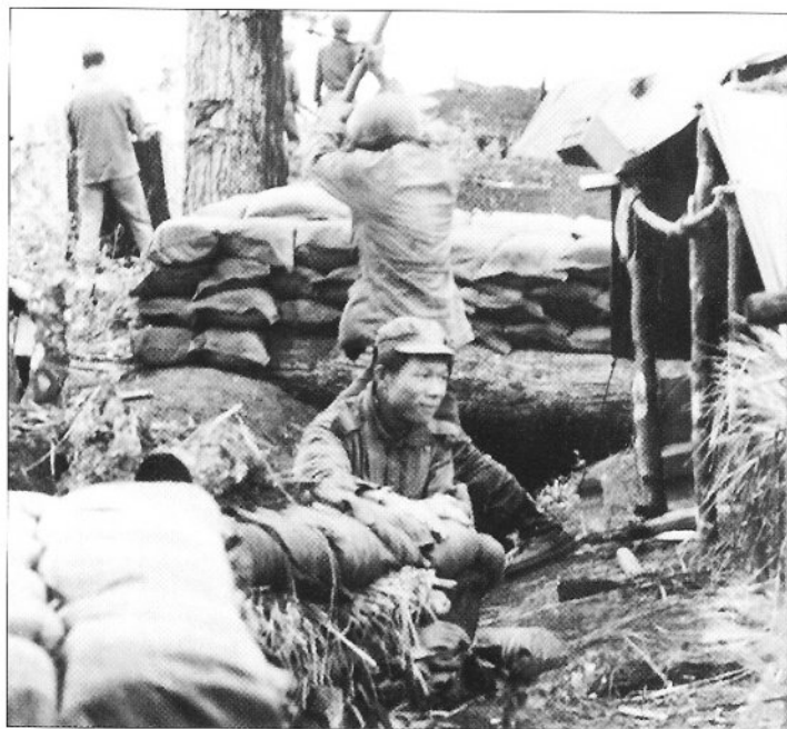
45th ARVN Artillery Regiment digging bunkers and trenches on commanding ground at FSB Mike Smith, 1970. Note the use of tree trunks in the constructions. This is yet another example of the way in which building materials had to be improvised and scrounged, since there were never enough ready-made construction elements provided from central stores. (US National Archives)
